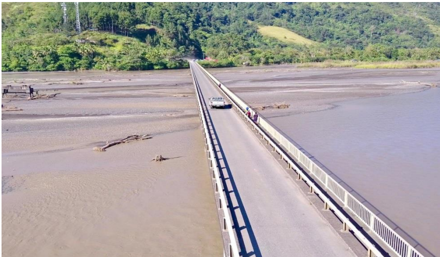
Existing Markham River Bridge near Lae
