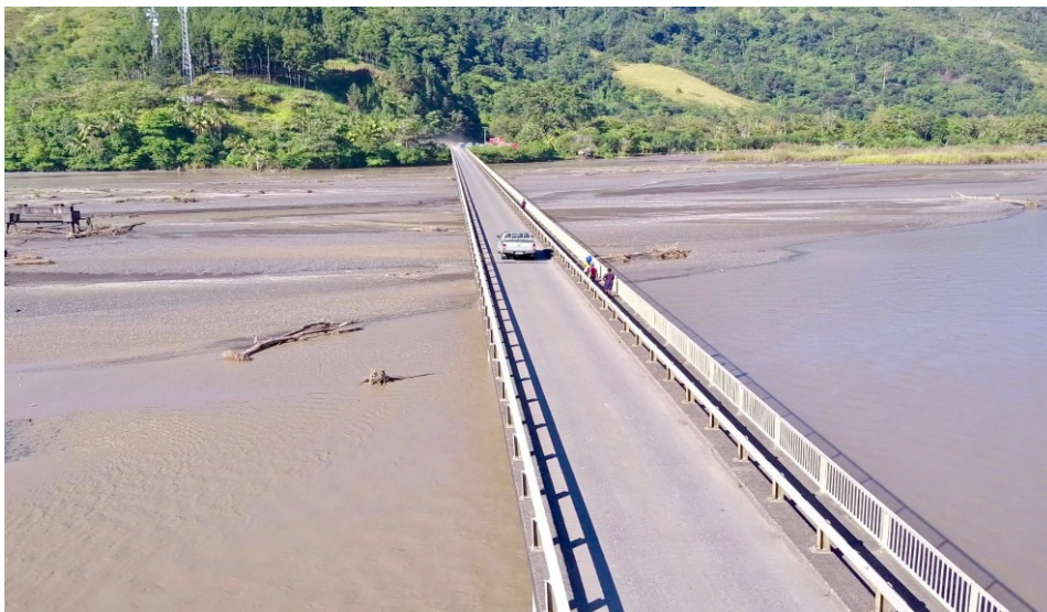
Existing Markham River Bridge near Lae
