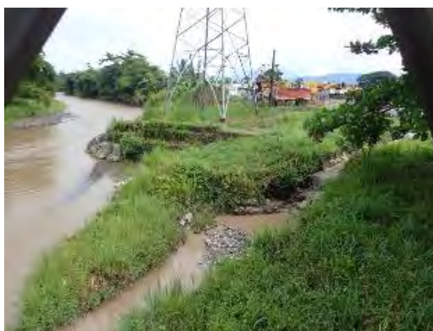
Plate 4.1: Open stormwater drain upstream of BUMB3
