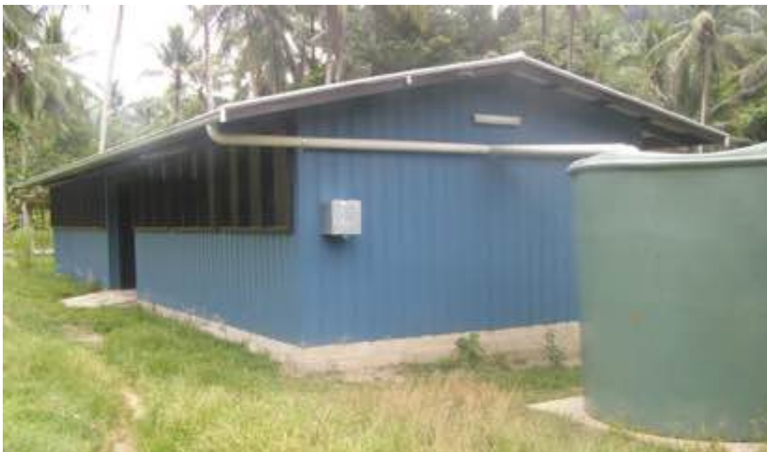
Plate 5.11: New elementary school at Pekumbe, March 2014
