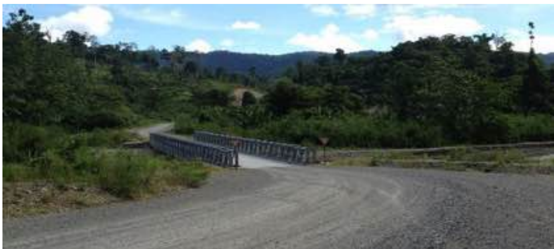
Plate 5.13: Bailey Bridge constructed in 2013 at Gingen
