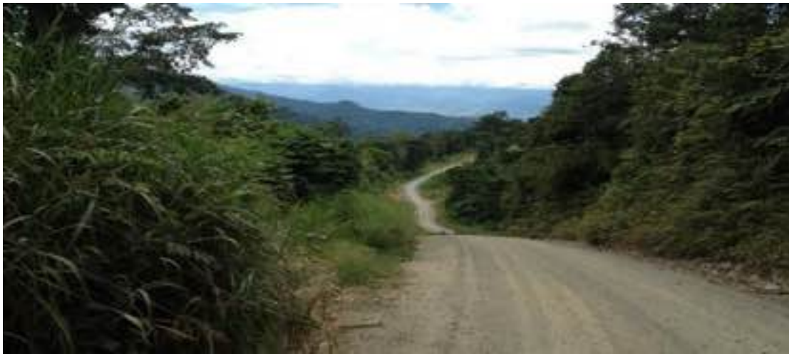
Plate 5.12: Undulating Demakwa Access Road
