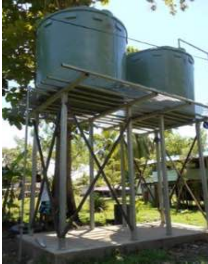
Plate 5.51: Water tower feeding communal tap stands at Wagang
