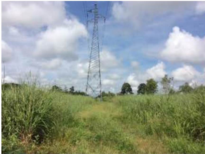
Plate 5.18: PNG Power transmission line corridor to be followed by Infrastructure Corridor near Zifasing
