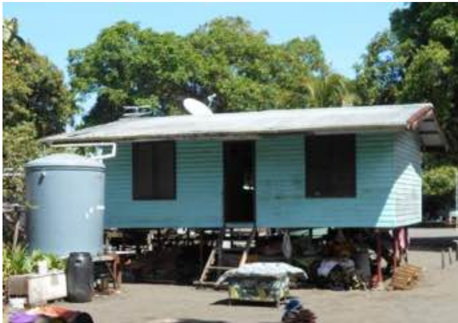
Plate 5.52: Rain tank installed at private home in Wagang
