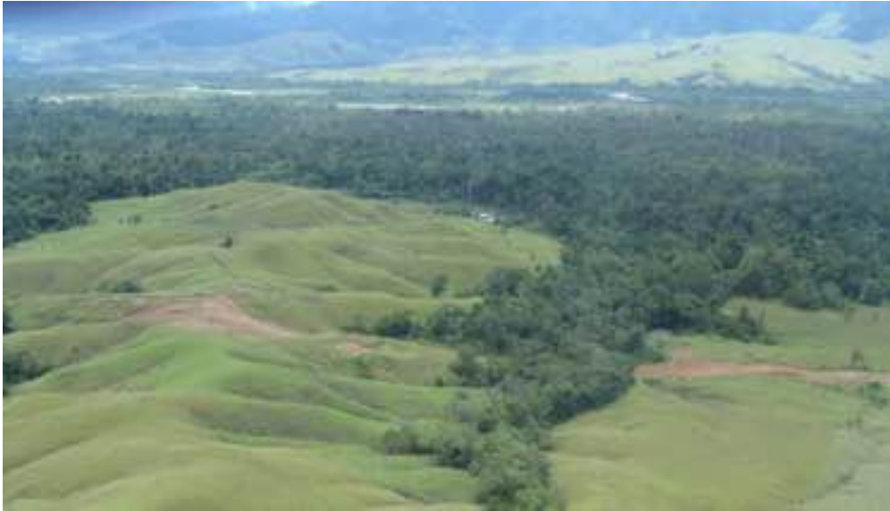
Plate 1: Proposed infrastructure corridor topography (Southern Section) including Mine Access Road (foreground) and Watut River floodplain (background) – view W
