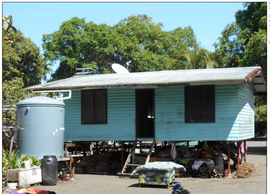
Figure 12.45 Rainwater tank installed at private home in Wagang
