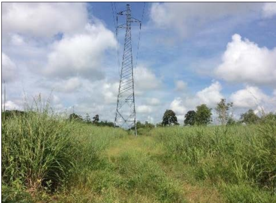
Figure 12.7 PPL transmission line corridor near Zifasing
