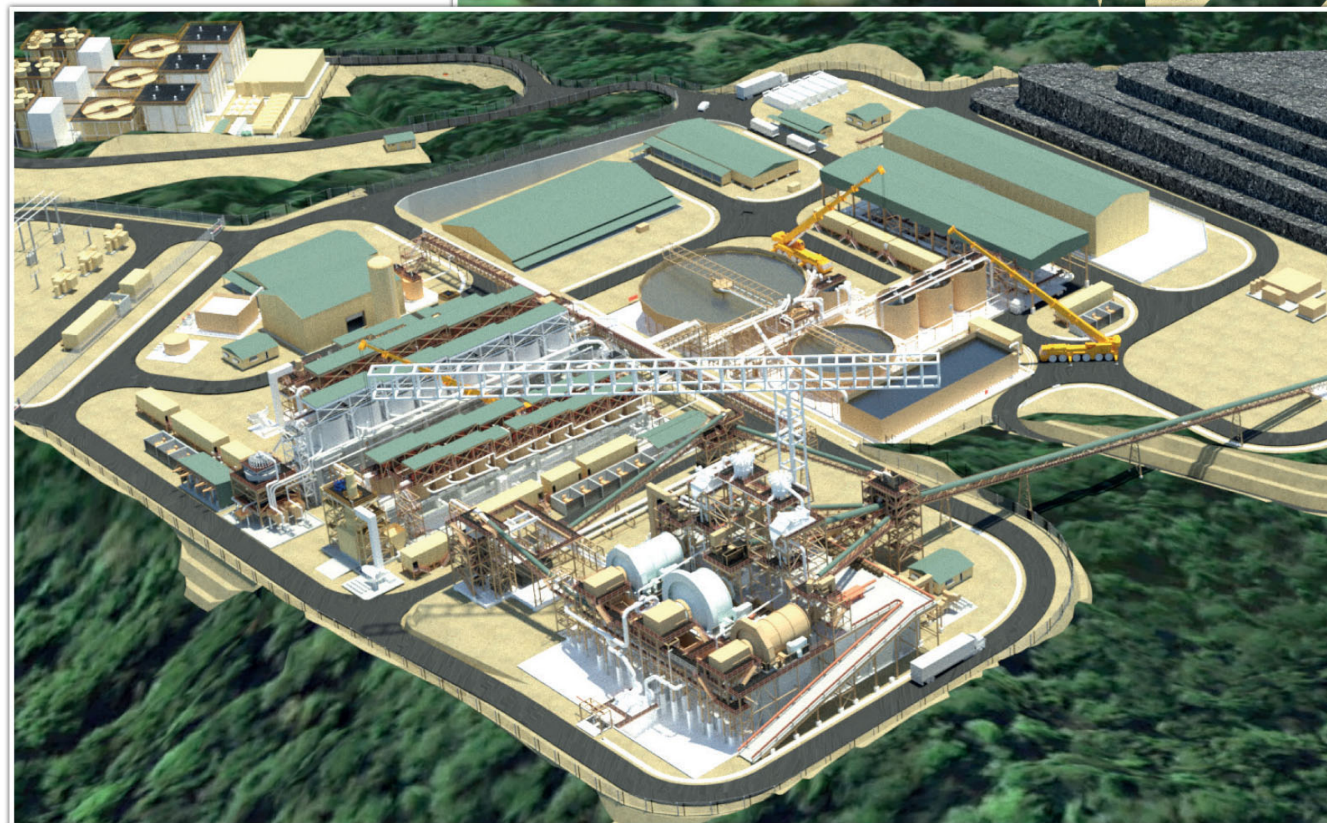
3D model showing process plant terrace and Watut portal terrace infrastructure (above) and flotation circuit (below)
